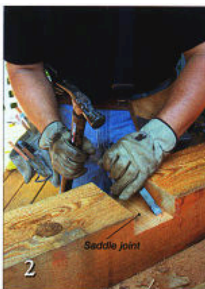
2 To cut the saddle joint where the center post and crossbeam meet, make repetitive passes with a circular saw, and remove the waste with a sharp chisel.
