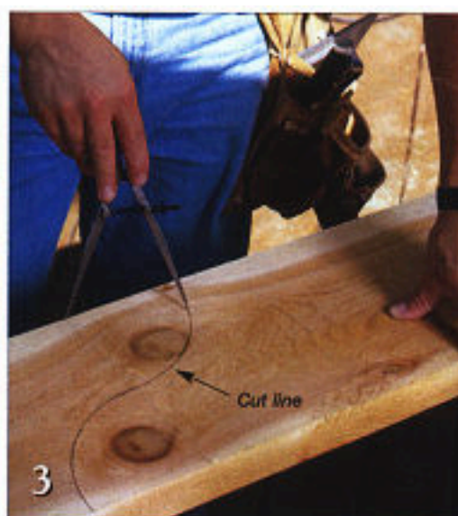
3 Scribe a decorative profile on the ends of the headers, ridge and rafters. There's no set rule to the design — just pick a profile that looks good to you.
