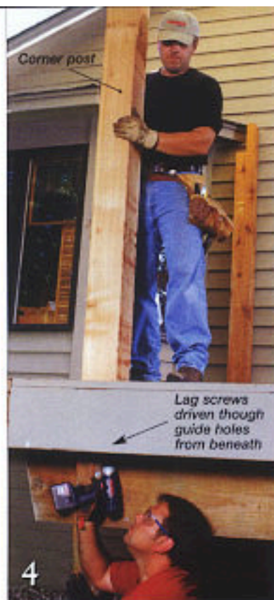
Hold the 6x6 posts in place and, from beneath, drive two 8-in. lag screws in each post. If necessary, add extra blocking after you've driven the screws.
