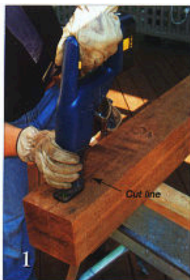
1 Cut a 4- x 10-in. notch in the top of each of the four 6x6 corner posts to support the doubled 2x10 full-size headers.
