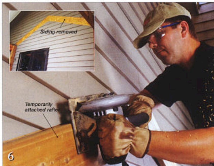
Temporarily attach the first rafters to the house, and use them as a cutting guide. Be careful to not cut so deep that you damage the sheathing beneath the siding. When the cuts are complete, take down the rafters and remove the cut siding.
