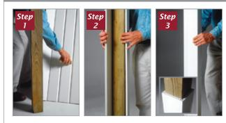
Simply apply adhesive in the joints of the column wrap.
