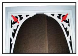
**Step 1**-Line the Windbreaker Panel frame up with where the screen section begins at the top of your screen door.
