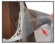
**Step 4-**Remove the protective film from both sides of the Acrylic Panel.
