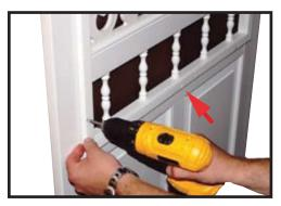
**Step 3** - Now drill in the provided screws into the bottom of the Windbreaker Panel frame (bottom 3 holes and sides).
