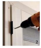
5) Open the non-operable door and extend the locks on the Astragal. Place a small amount of caulk onto the Astragal locks. Close the door again and once in place, extend the locks. This will mark where you need to drill for the locks. Using a 7/23 drill, drill the holes where marked.
