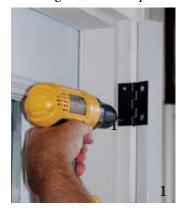
4) Once the Astragal has been notched (if necessary), slide the operable door into the other hinge bar. Close both doors, space the door and or Astragal as necessary, attach the Astragal and hinge bar with screws provided.
