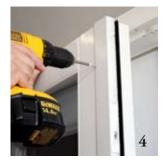
2) Once the bars are mounted, slide the door that is to be the non-operable door into the Hinge Bar. Place the door in a closed position to square the door and attach the Hinge Bar with 3 screws.
