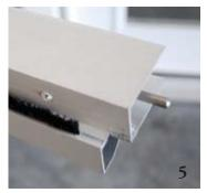
ch Door 3) Slide the Astragal over the door, the weather strip should be out. Close the door to determine if the Astragal needs to be notched.
