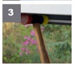
Install screen using retainer strip and rubber mallet to outside portion of porch
