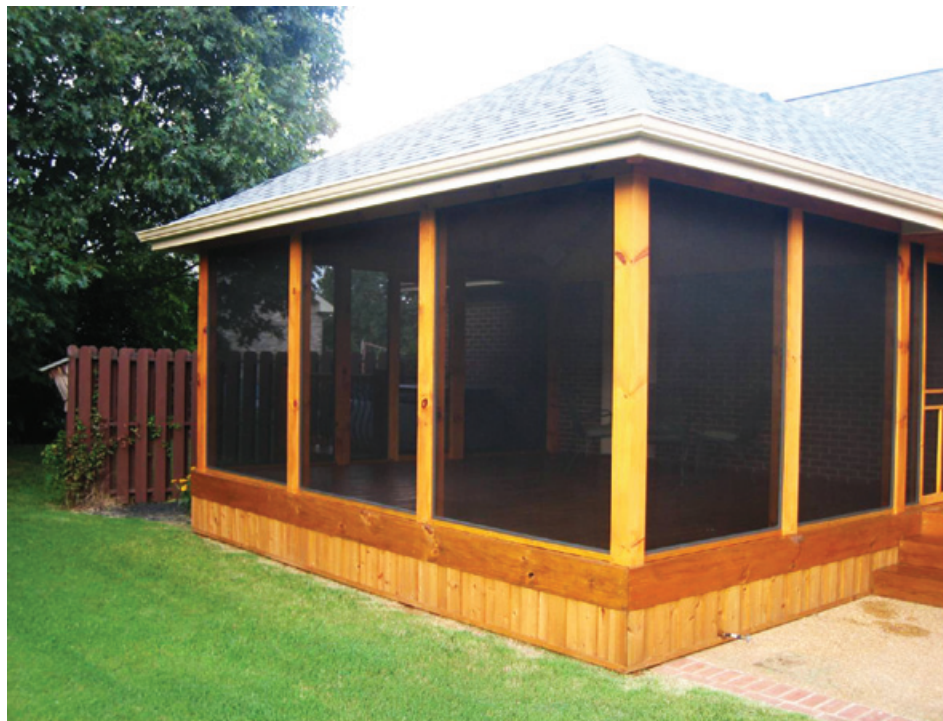
Mt. Juliet, TN homeowner Brett Keiper recently installed the MINI Track™ porch screening system from Screen Tight™ on the back of his 2,200-square foot brick ranch house.
