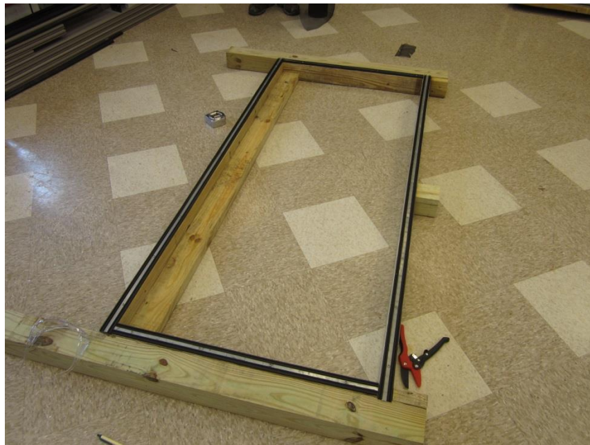
Photo No. 4 Railing Assembly Prior to Installation of Screen
