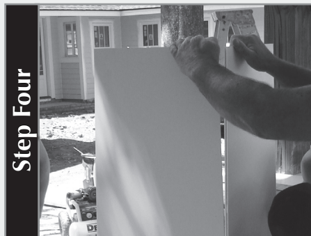
Step Four Snap remaining 2 Tapered Panels together after applying small bead [1/16"] of PVC adhesive in groove, thus forming 2nd half. [Note: An excessive amount of adhesive in the snap lock may result in a sink line in the outside surface.]
