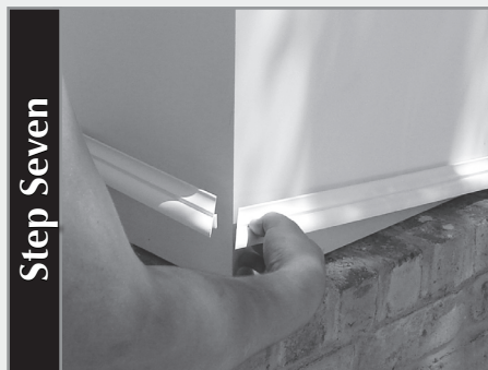
Step Seven Attach Bead Molding Trim by snapping ends together around existing column. Optional to glue or nail in place.
