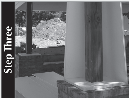
Step Three Snap 2 Tapered Panels together after applying small bead [1/16"] of PVC adhesive in groove. Set 1st half of column in place against Squaring Blocks. [Note: An excessive amount of adhesive in the snap lock may result in a sink line in the outside surface.]
