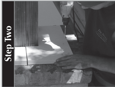
Step Two Attach the top and bottom squaring blocks with appropriate fasteners.
