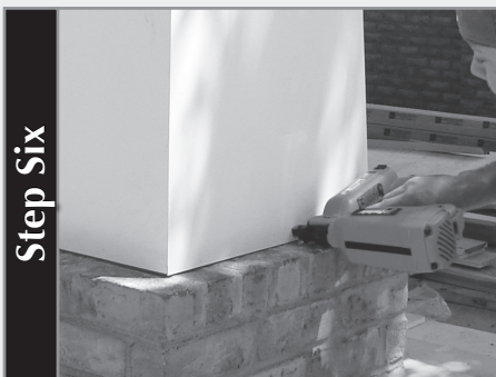
Step Six Fasten top and bottom of Tapered Panels to squaring blocks with rust resistant nails.
