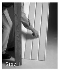
**Step 1** - Handle Column Wrap with care to prevent the joint tape from tearing. Cut Column Wrap to proper height. Apply a bonding adhesive inside each groove. A 1/8" bead along the total length is recommended in the mitered corners. A 1/16' bead is recommended in the snap lock. (Note that an excessive amount of adhesive in the snap lock may result in a sink line in the outside surface.) For optimum results, use and adhesive with moderate setup time.
