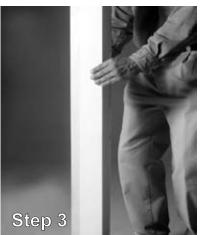
**Step 3** - Once the bonding adhesive has set-up - *typically a 24-hour period* - remove the temporary joint tape and your column is complete.
